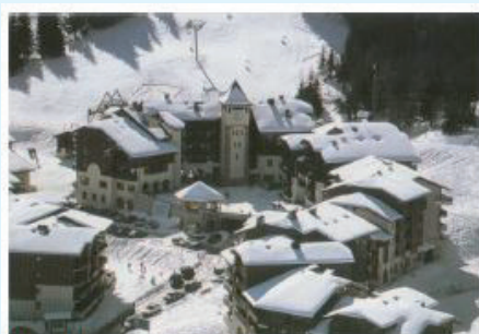
Station des Esserts
